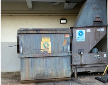
Hall Towers Compactor
